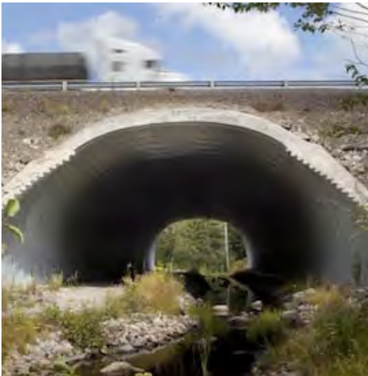
Open Bottom Culvert along the Trans Canada Hwy, Banff
