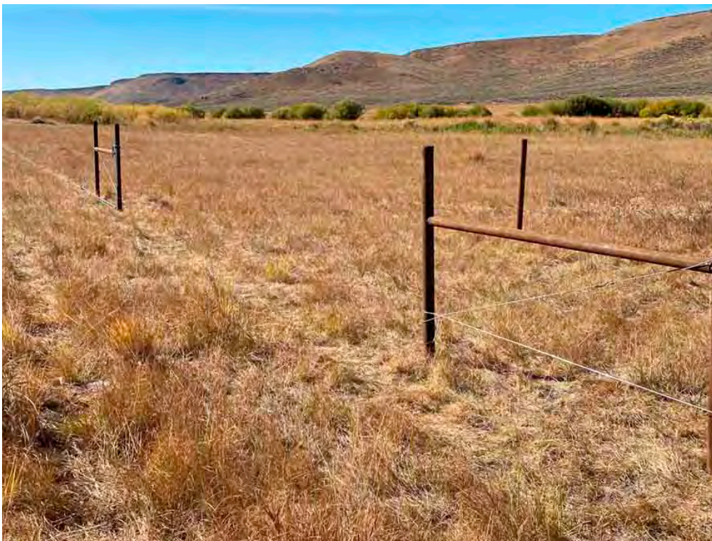
Metal H-brace Ready for Lay Down System
