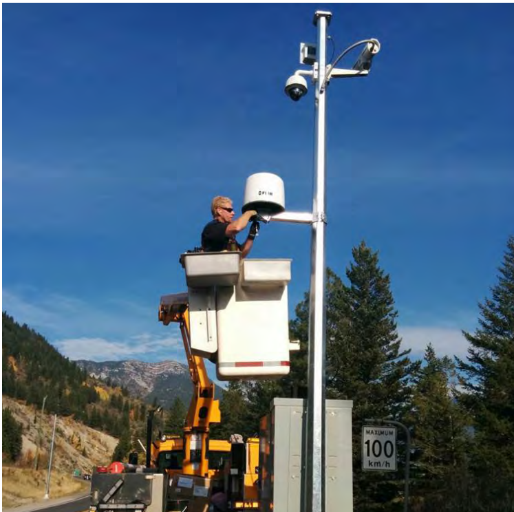
Animal Detection System on Highway 3, Alberta, Canada
