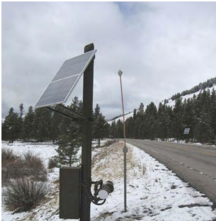
Animal Detection System on U.S. Highway 191 in Yellowstone National Park
